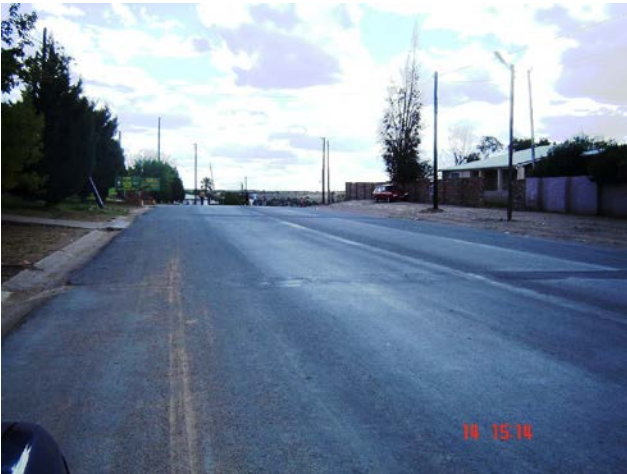
Old patch areas and existing canals
