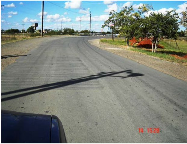
Concrete widening on curve
